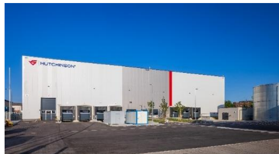
Mannheim Distribution Center ©Goldbeck
